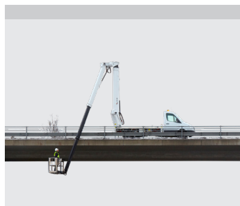
Ability to work below ground level (-3,3 meters)
